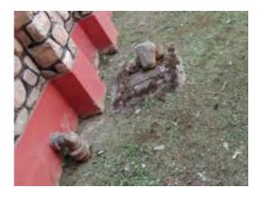
Figure 18: Foundation Exploration of Masonry Block
