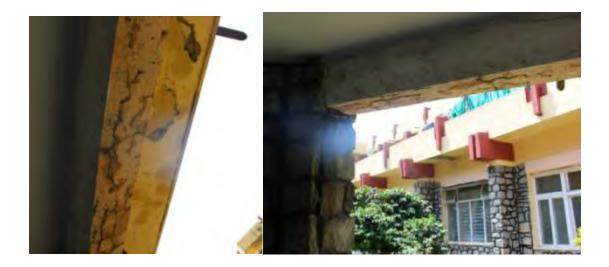
Figure 5: Corrosion cracks in Emergency Block & OPD Block
