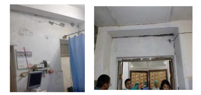
Figure 9: Pounding Effect at ENT and CT Scan Block Connection
