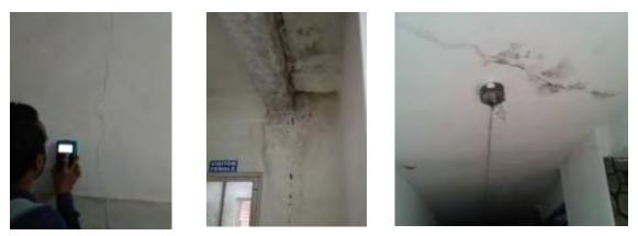
Figure 8: Vertical Cracks on Masonry Wall (Sealed area of Seismic Separation)
