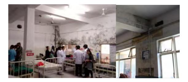
Figure 4: Serious seepage issues inside Emergency Block & OPD Block
